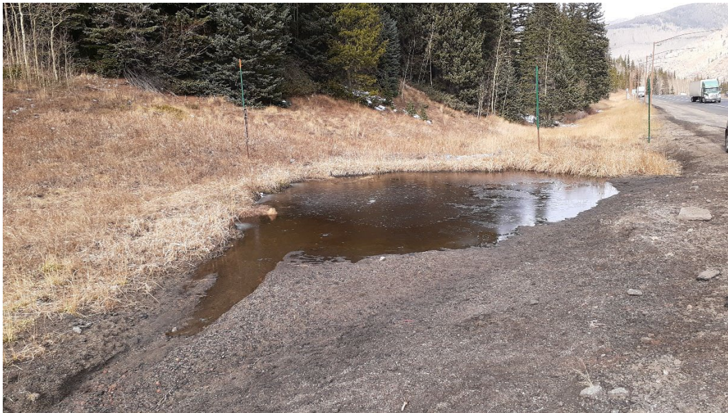
Figure 3.1 Soft-sided Sediment Basin No. 30 on Eastbound I-70
