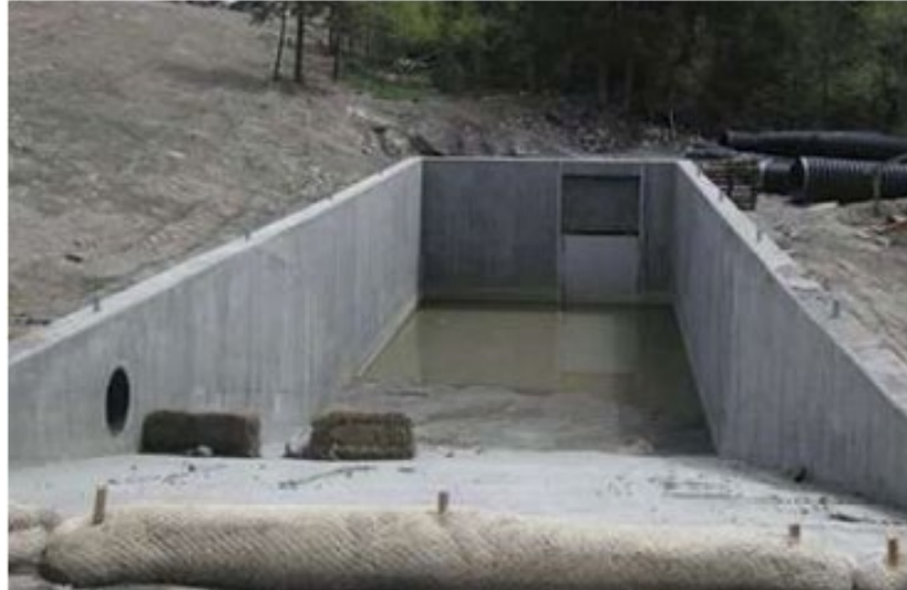
Figure 3.4 Loading Dock Trap (Berthoud Pass East)
